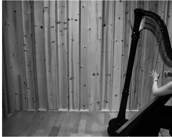
Figure 10.5 A home built diffusive wall randomly scatters reflections, reducing standing waves while opening up the sound of the room, and keeping it relatively bright.
