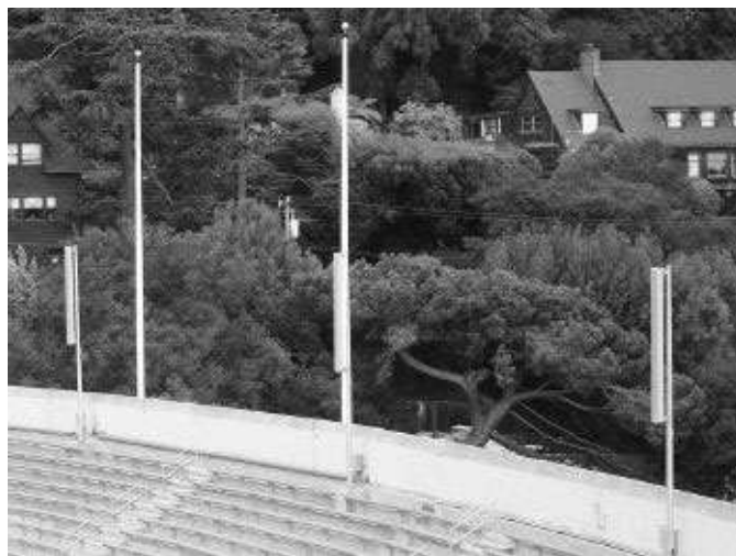
Figure 11-17. Distributed column loudspeakers mounted at back
