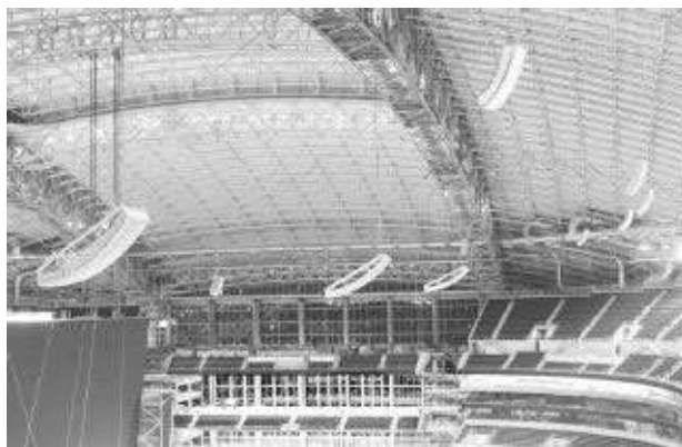
Figure 11-19. Retractable roof stadium showing locations of distributed line array clusters.
