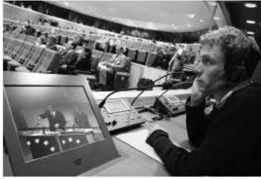
Figure 45-5. A fixed installation interpreter's booth showing three interpreter stations. Courtesy Listen Technologies Corporation.
