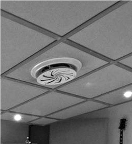
Figure 7.10 Nailor Industries Series RBD round diffuser. 3,5
