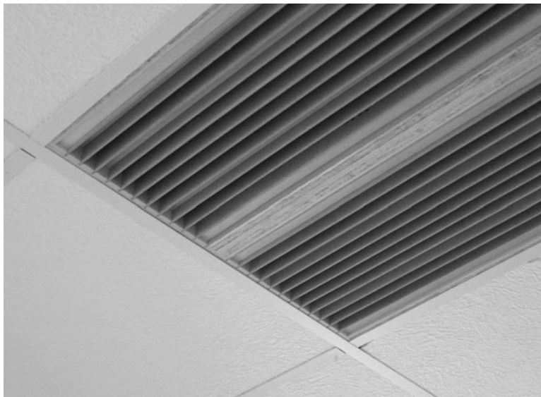
Figure 9.20 PI324 Quadratic Residue Diffusor in ceiling grid.
