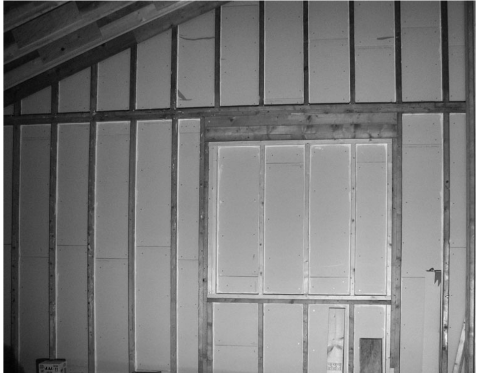
Figure 10.18 Exterior wall isolation.
