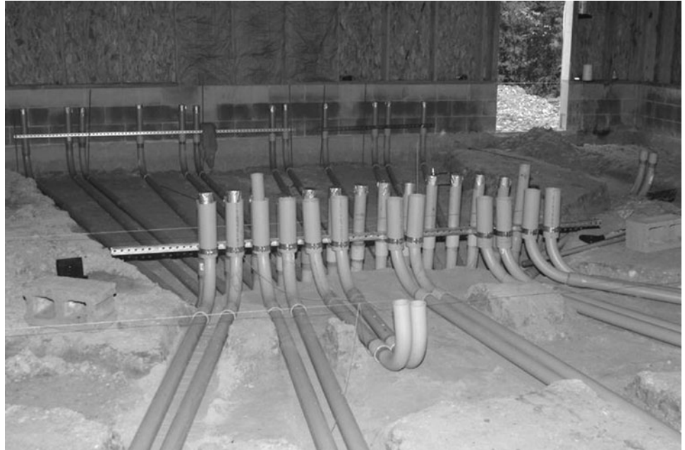
Figure 6.3 1 Low-voltage conduits.
