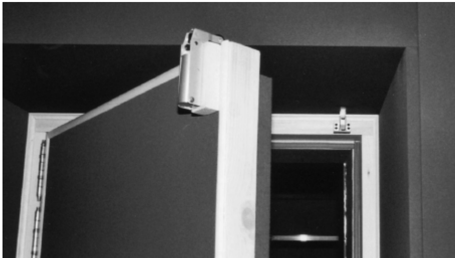
Figure 8.18: The hydraulic brake on the door engages with the hook on the frame when the door is closed. A hydraulic damper controls the rate at which the door can close the last few centimetres (as the roller on the brake is forced vertically upwards by the shape of the hook). Once 'over centre' the hydraulic ram works in the opposite direction, forcing the roller upwards and maintaining the door tightly closed.
