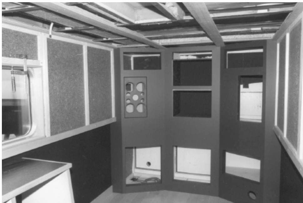
Figure 23.4: The basic framework of the Banzai monitor wall, with the lateral membrane absorbers also visible.
