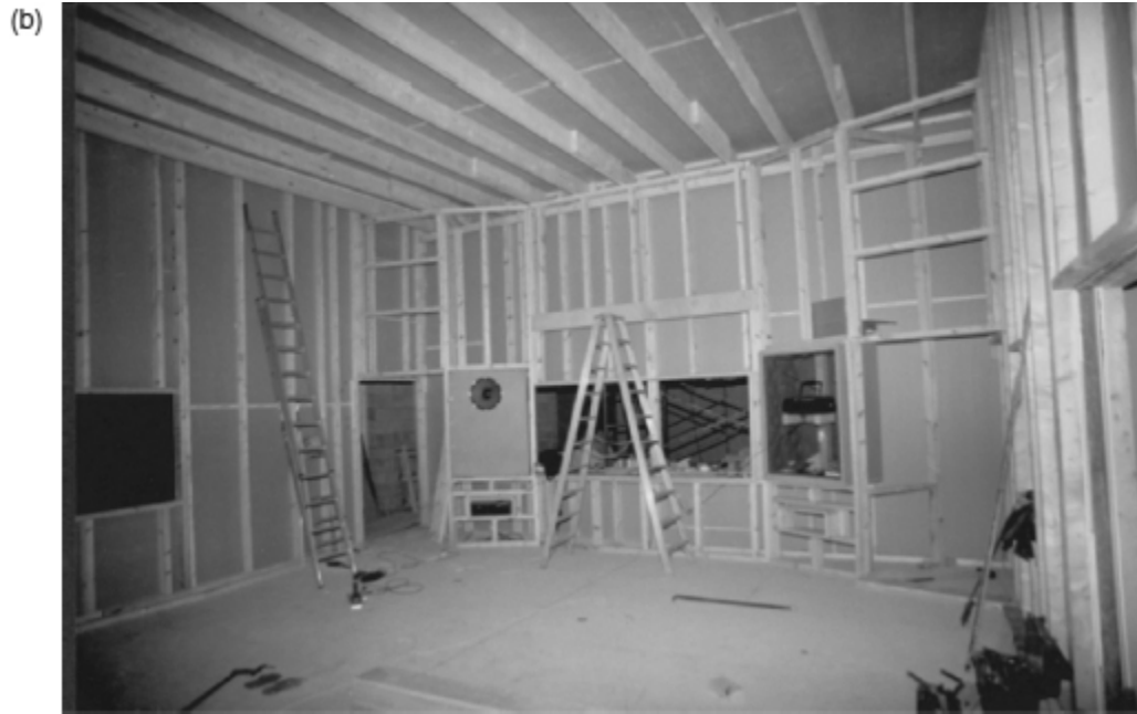
Figure A.1.9: (b) The loudspeaker wall framing at the stage of Measurement No 3.
