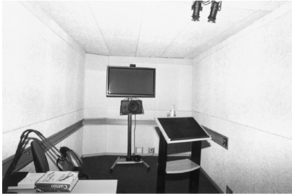
Figure 5.26: A room similar to the one shown in Figure 5.24 but after treatment with a more appropriate combination of materials, yet still only occupying the same space as the original panels (Sodiner, Vigo, Spain).
