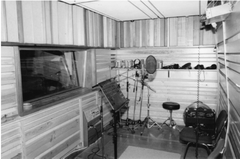
Figure 7.12: A vocal room where an attempt had been made to use a rotating panel system, as shown in Figure 7.9 , but with inadequately-sized panels and over an inadequate area of the room. The panels could only remove a little of the boxiness from the sound. They were more cosmetic than acoustically effective.
