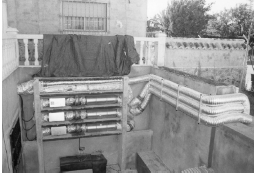
Figure 9.1: The ventilation system of a studio with three rooms. On the shelves are, from left to right, the filter boxes, the axial inline fans, and the 90cm long silencers. All the flexible ducting is of the acoustic type, which itself acts as an in-line silencer, except for the extensions on the outlet ducts to the right, which are simple, flexible aluminium tubes. The air inlet is where the cable tubes can be seen, at the bottom left of the picture. Normally, to comply with building regulations, the inlets and outlets should be at least 5m apart, to prevent recirculation of exhausted air. Audio Record Studios (now 'El Estudio de Domi), Morón de la Frontera, Spain (2001).
