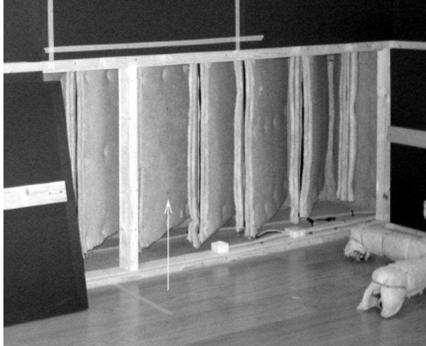
Figure A.1.17: The panel array behind the final, fabric covering.
