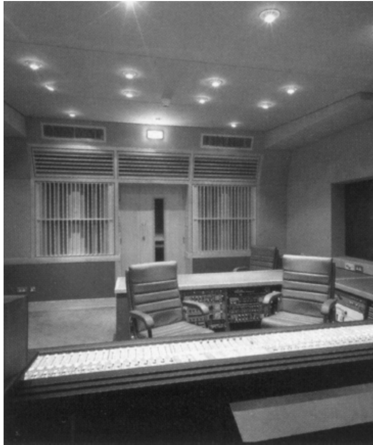
Figure 17.2: Rear end of a ‘Live End-Dead End’ room showing the diffusers. BBC, Maida Vale.
