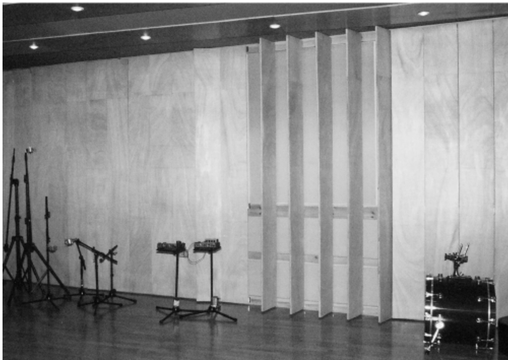
Figure 7.10: Multiple, hinged panels covering a large, full-range absorber. These provide considerable variability to the acoustics of the room. The different combinations available are almost infinite – Rockaway Studios, Castellón de la Plana, Spain (2008).
