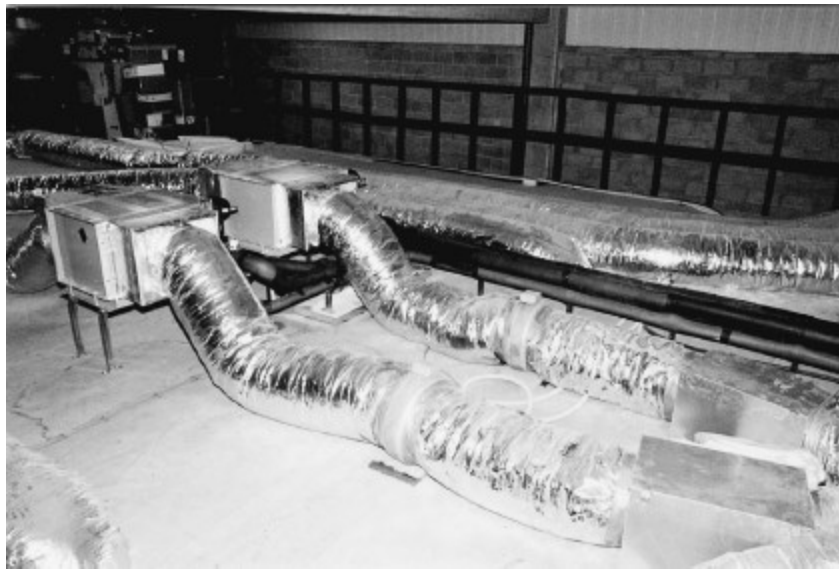
Figure 9.4: In the system shown, the air enters through the rectangular filter boxes on the extreme right of the photograph, before passing through the fans. The heat exchangers are the large rectangular boxes, fed with water via the black insulated pipes.
