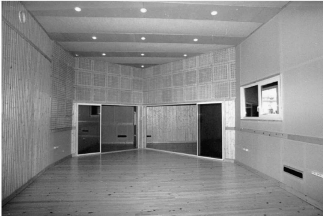
Figure 7.1: Dobrolet Studio, St Petersburg, Russia (1996). Note the ex-Soviet era perforated diffusers over the glass doors and on the adjacent left-hand wall.
