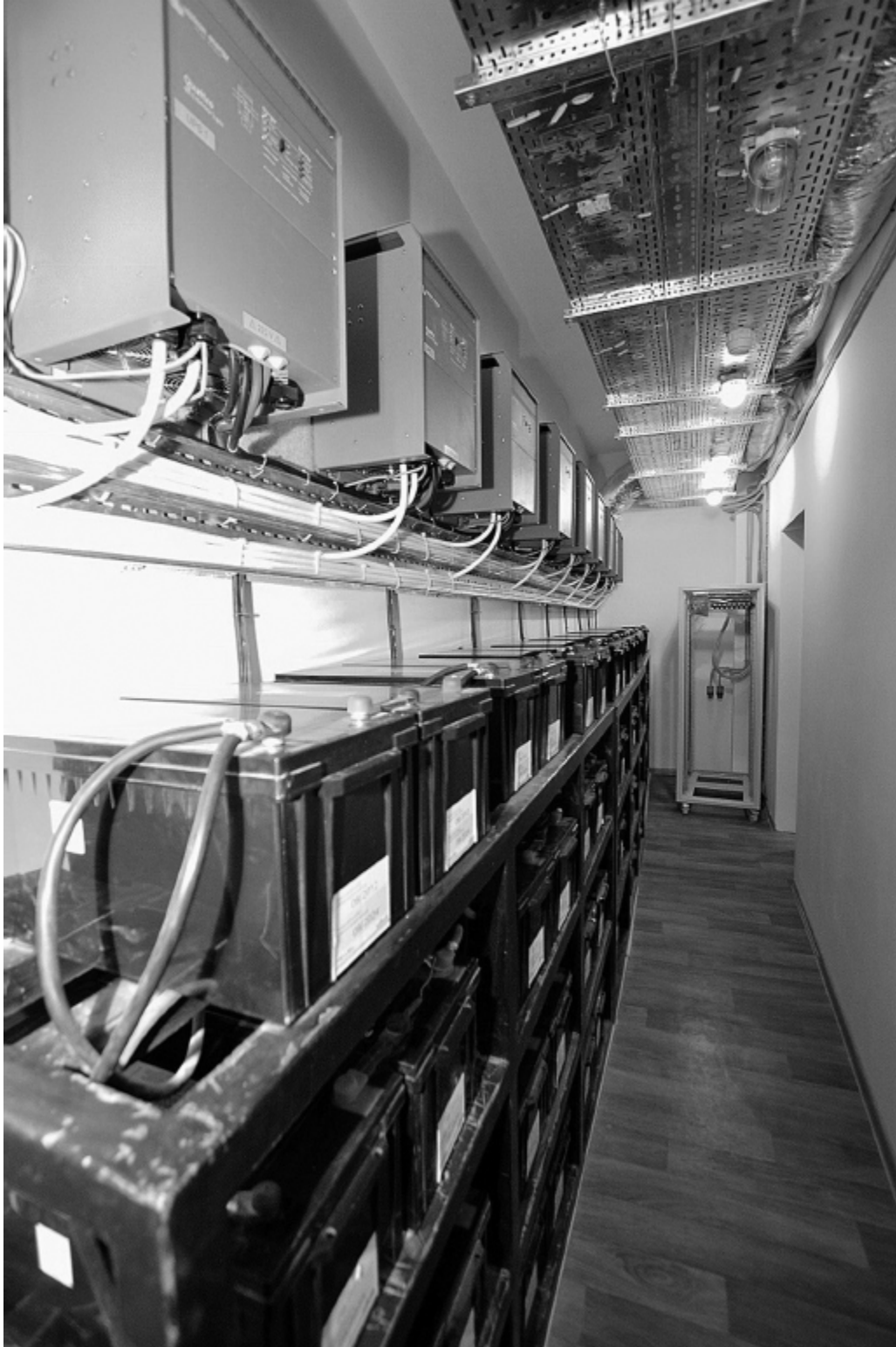
Figure 25.8: The back-up-power room at NTV-Kino, in Moscow. The row of parallel-connected, Victron inverters can be seen attached to
